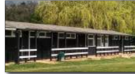
The newly painted Westwood Park pavilion
